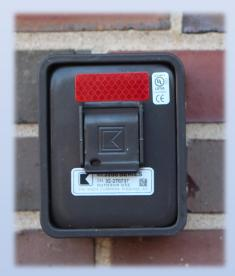
A Knox Box is a secure key safe that mounts on the wall of a building near the entry door. The only keys available to open the Knox-Box are in the possession of the fire department.
